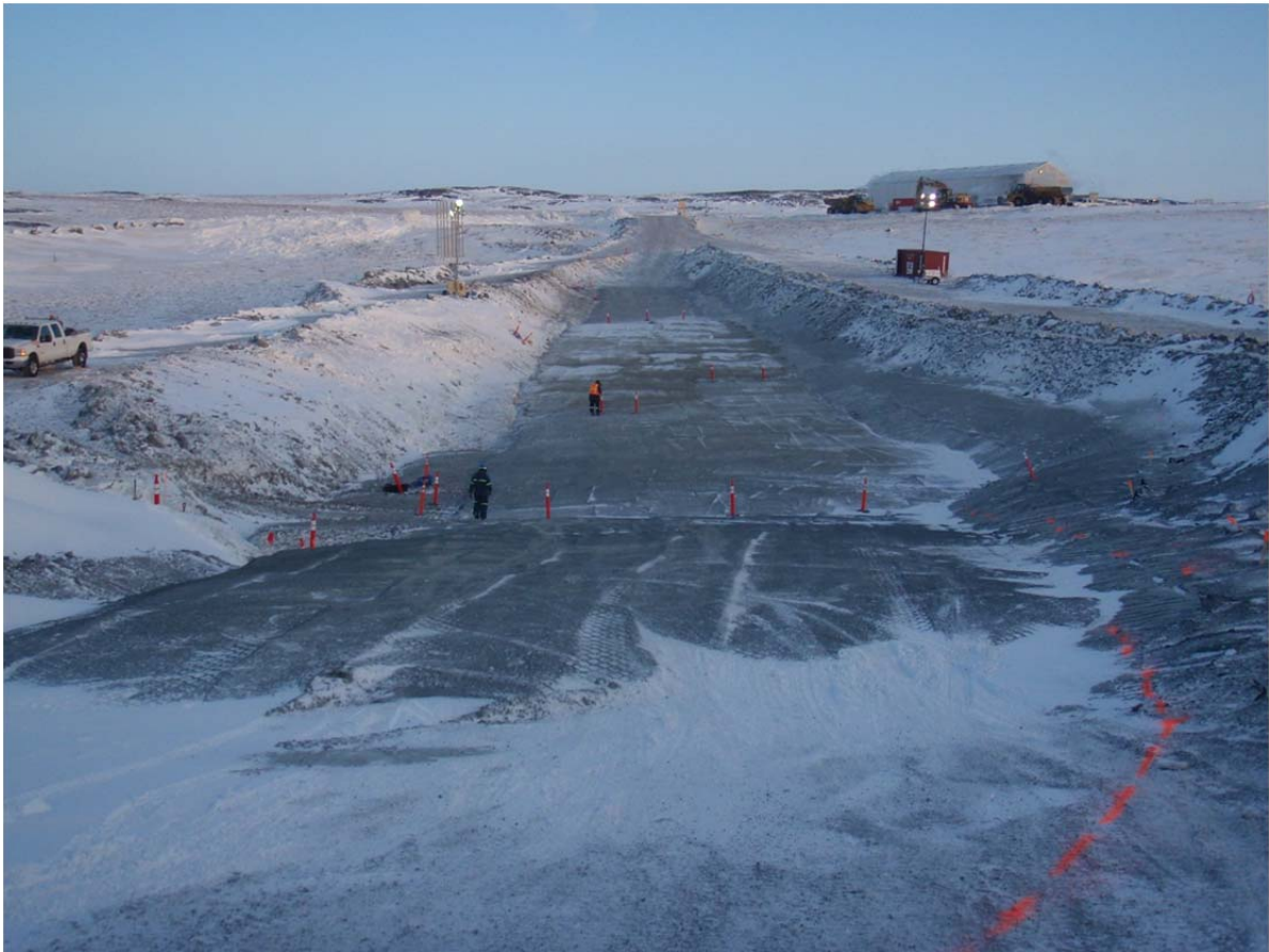
Photo 1: ~NE view down keytrench. Note the area to the East (towards the FCP) of the closest set of delineations is the area where FCM was placed on Jan 27 th .
