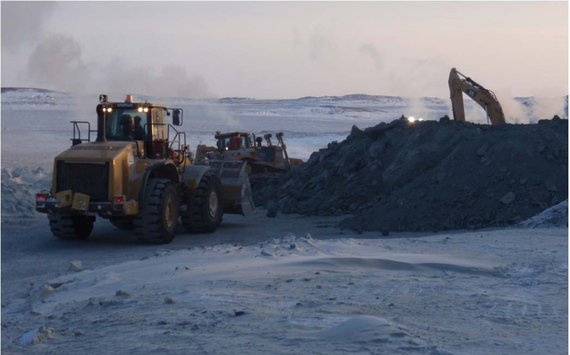
Photo 6: ~ESE view of the loader, D8 dozer and 345 excavator working on breaking up the unsaturated FCM stockpile at the FCP Pad.
