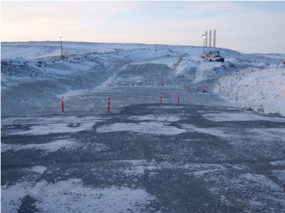
Photo 3: ~ WSW view down key trench from ~ station 1+40. Looking over FCM placed on Jan 27 th .
